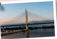
A cable-stayed bridge has one or more towers with cables that run from the tower to the deck. The cables support the deck of the bridge.
